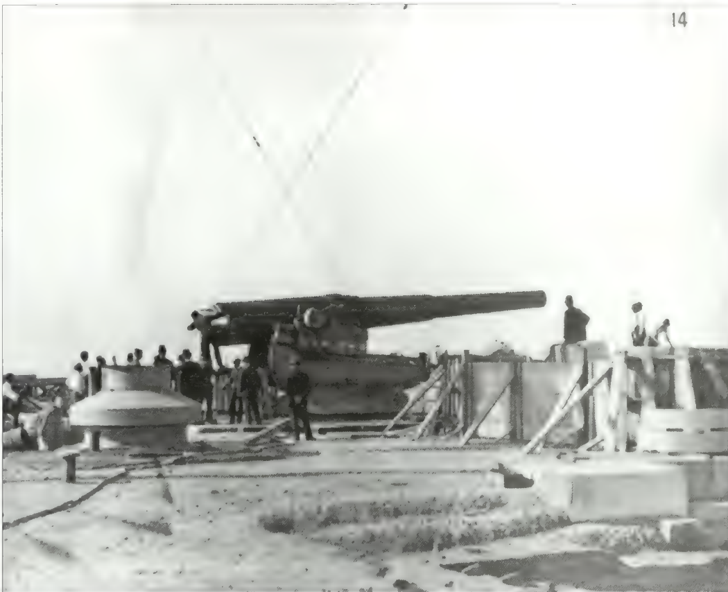
Figure 2.15. Battery Potter's north emplacement, September 12, 1892. The first of Battery Potter's two 12-inch guns was mounted at the north emplacement in August 1892. A month later, two rounds were test fired inaugurating a new era of coastal defense for metropolitan New York (GATE 7804).
